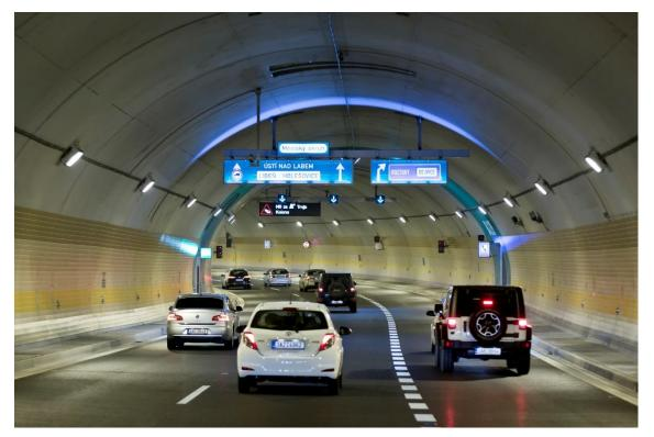
Picture 10 – pre-signalling of an exit (first place) - signalling of an escape with blue underlining (second place) - VMS with the information of a traffic jam (third place.)
